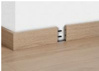
Connection of 2 skirting boards along the wall
